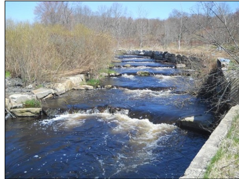
Photos of Riffle and Pool design on the Acushnet River.
