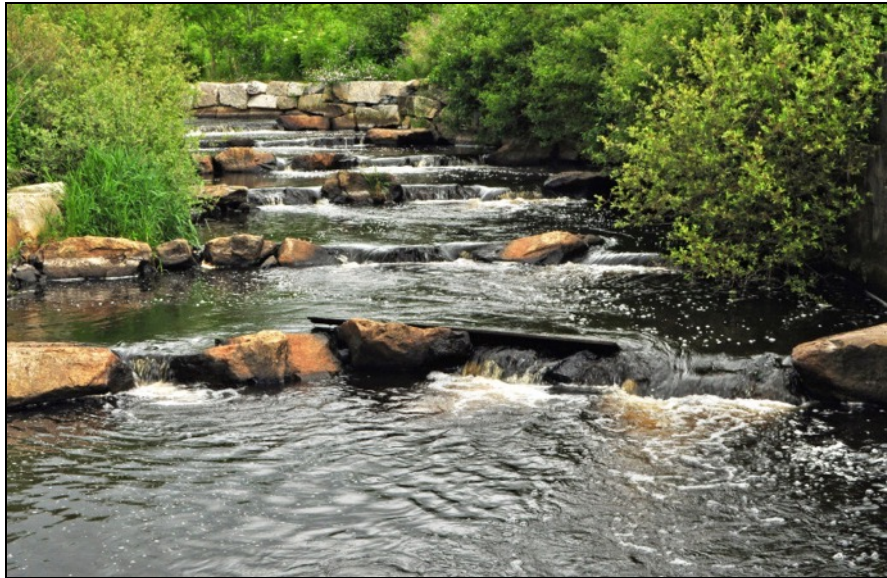
Photos of Riffle and Pool design on the Acushnet River.
